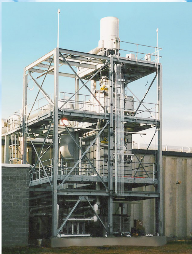
20,000 CFM Wet ESP for submicron particulate removal from oven exhaust at a textile plant
