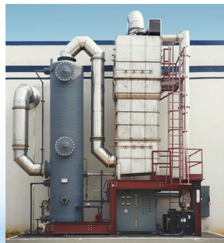
5,000 CFM Multi-Stage Scrubber System with FRP acid gas scrubber and 317SS Wet ESP
