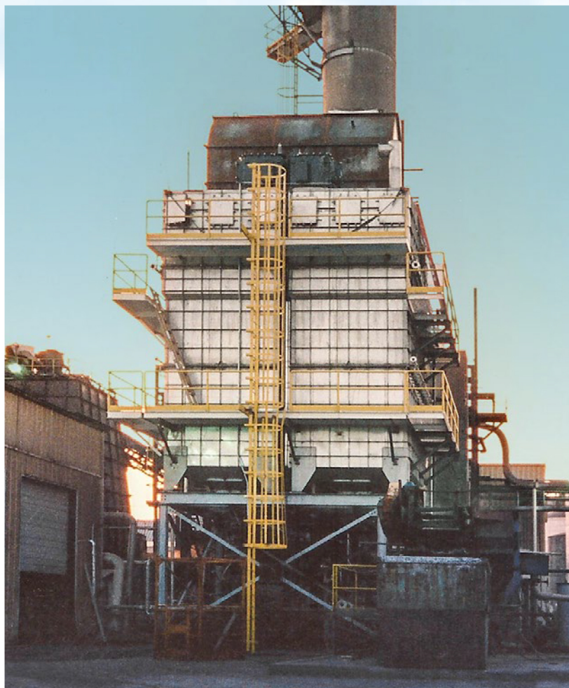
120,000 CFM Wet Electrostatic Precipitator treating waste fuel boiler emissions at a paper mill
