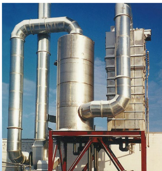
6,000 CFM Wet ESP and gas scrubber installation
