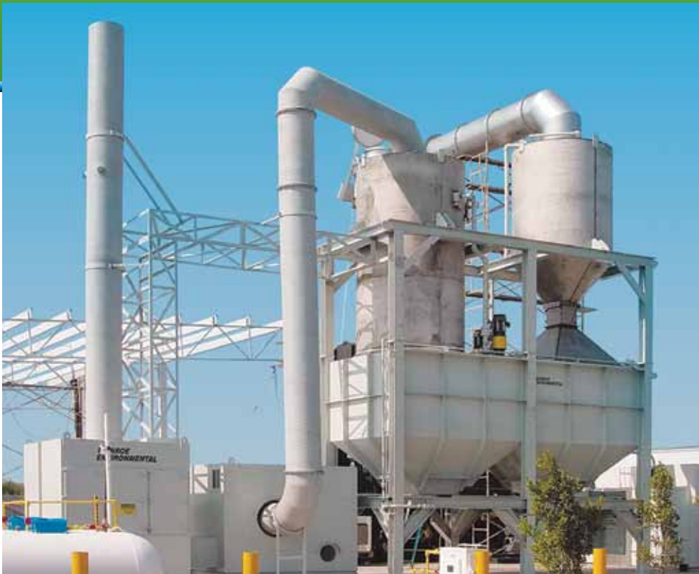
20,000 CFM Multi-Stage Scrubbing System for solid waste incineration process. (From right): Ceramic-lined inlet duct, rapid water quench, adjustable Venturi Scrubber, liquid clarification tanks, Packed Bed Scrubber, and Carbon Adsorber.
