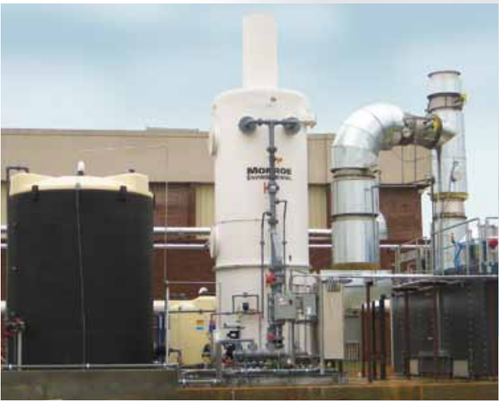
12,500 CFM Packed Tower Scrubber removing SO 2 and Cl 2 from regenerative thermal oxidizer (RTO) exhaust
