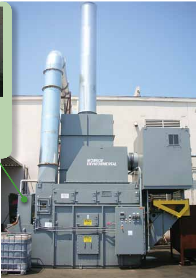
Oil Recovery Unit (Belt Skimmer) continually recovers condensed grease from scrubbing process
