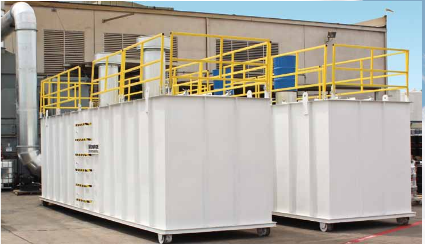
(2) 15,000 CFM Deep Bed Carbon Adsorbers, mild steel construction with specialty exhaust stacks for odor control at a grease manufacturing facility
