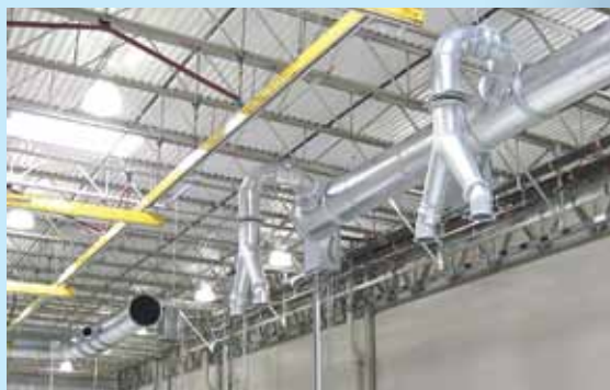
Tapered ductwork system with individual source hoods for multiple Oil Mist Collectors on a high production machining line
