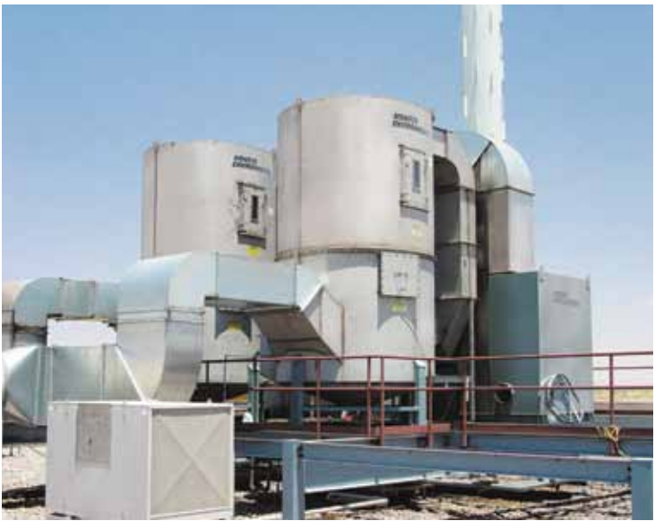
25,000 ACFM Scrubbing System at a textile plant to remove particulate and acid gasses
