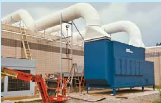
Custom designed ductwork system with supports for recirculating climate-controlled clean air after filtration through a 30,000 CFM Oil Mist Collector
