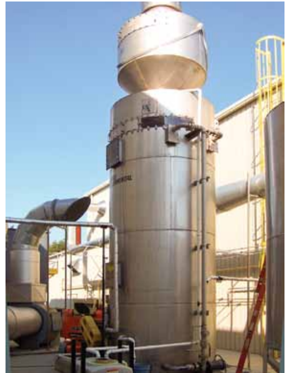
15,000 CFM Packed Bed Scrubber to remove ethylene glycol and NMP fumes from a glass coating operation
