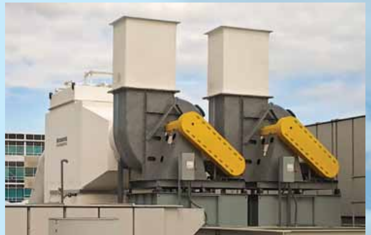
Chemical Storage Tank Vapors: 30,000 CFM Horizontal Packed Bed Scrubber with polypropylene construction to remove chemical fumes emitted from acid-dip tanks at a semiconductor manufacturing facility. Dual-train exhaust ductwork with automated dampers and FRP fans provides maximum control over the scrubbing process.
