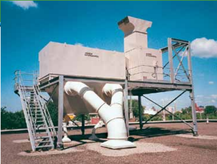
20,000 CFM Dust Collector, roof-mounted with stairway and access platform
