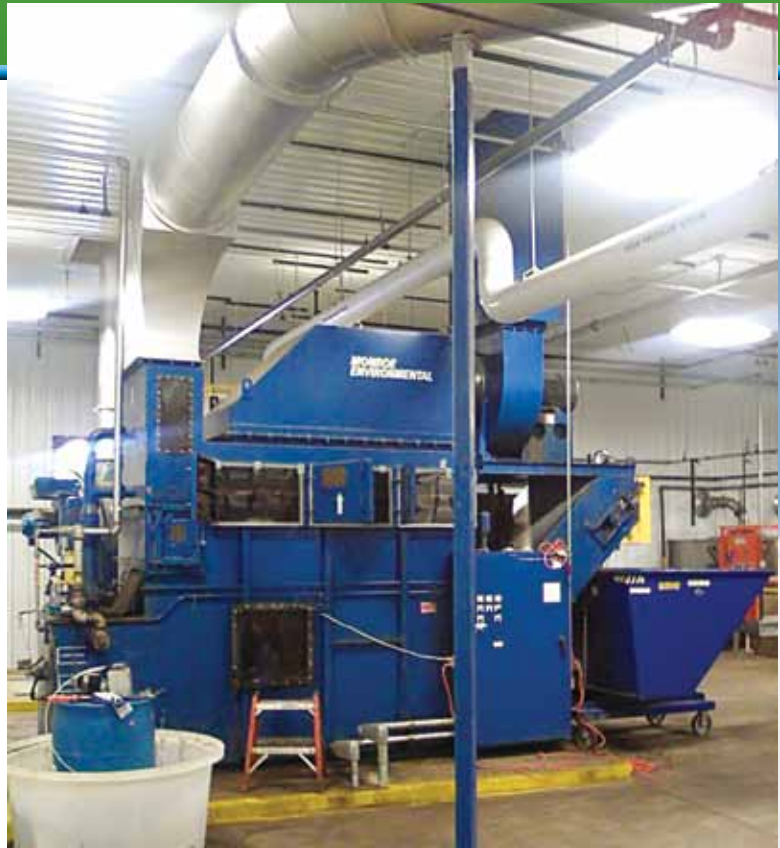
9,600 CFM Dual Throat Venturi Scrubber for removal and recovery of fly ash from the exhaust of a wood fired boiler
