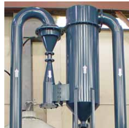
Fixed throat Venturi Scrubber followed by cyclonic separator for a lime dust scrubbing process
