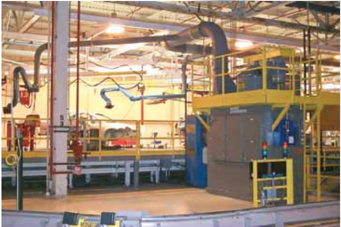
9,000 CFM Mist Collector for an automotive paint spraying operation
