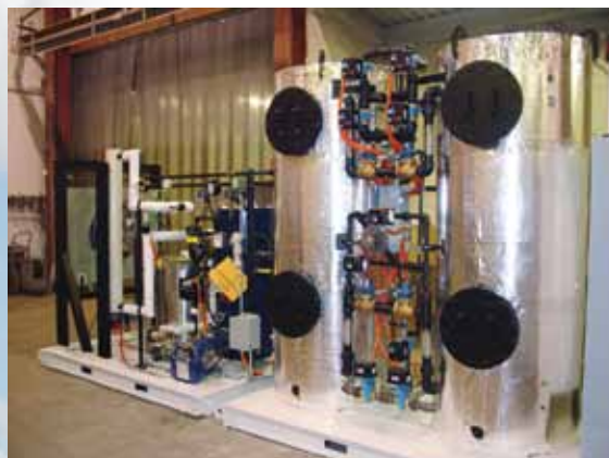
High pressure scrubbing system to remove sulphur compounds from a propane gas supply
