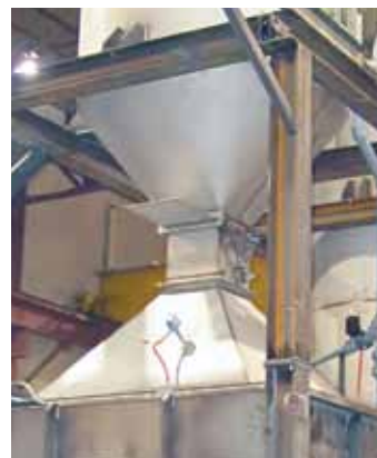
Adjustable, rectangular Venturi Scrubber throats for wet dust collection
