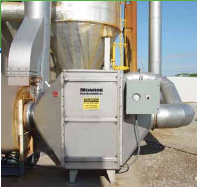
10,000 CFM Multiple Tray Carbon Adsorber, stainless steel construction for odor control at a grainery
