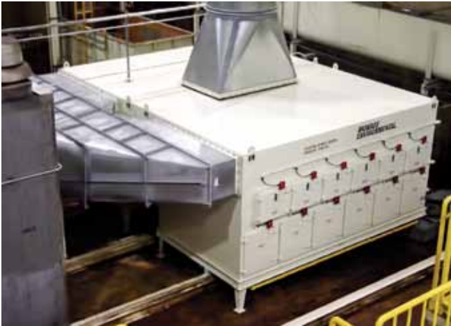
50,000 CFM Oil Mist Collector with custom ductwork and airflow monitoring system
