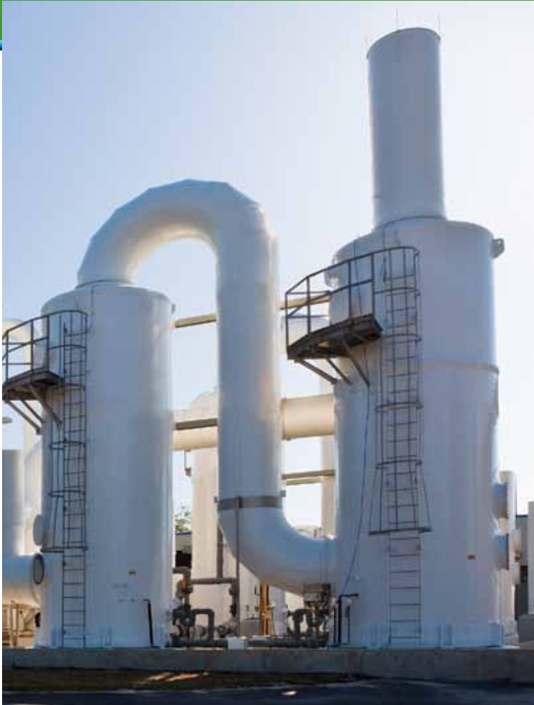
Municipal Treatment Plant Odors: Hydrogen sulfide ( H_2S ) and ammonia ( NH_3 ) odors that are common at municipal water and wastewater treatment plants can be efficiently targeted and removed by a Multi-Stage Packed Bed Scrubbing System.
