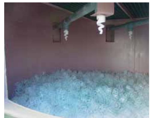
Non-plugging spray nozzles above bed of loose fill polypropylene packing
