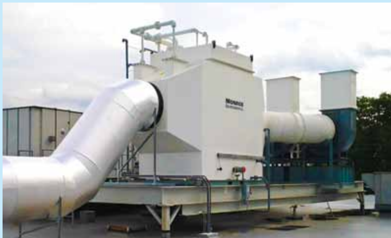
Chemical Storage Tank Vapors: 30,000 CFM Horizontal Packed Bed Scrubber with polypropylene construction to remove chemical fumes emitted from acid-dip tanks at a semiconductor manufacturing facility. Dual-train exhaust ductwork with automated dampers and FRP fans provides maximum control over the scrubbing process.
