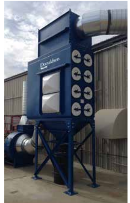
DFO on Plastics Routing 16,000 cfm (27,184 m 3 /h)
