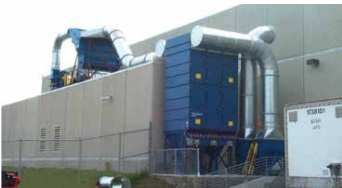
DLMC on Paper Dust 27,000 cfm (45,864 m 3 /h)
