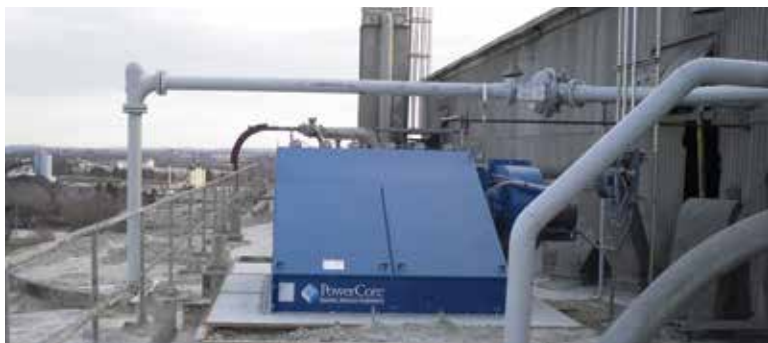
CPV - Multiple Cement Silos 4,800 cfm (8,154 m 3 /h)
