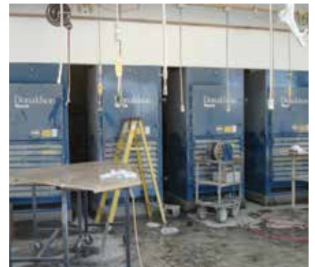
DWS on Granite Finishing 22,000 cfm (37,370 m 3 /h)
