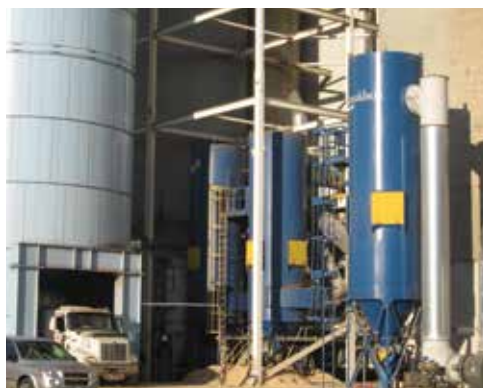
RF - Grain Terminal 34,000 cfm (57,754 m 3 /h)
