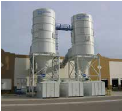
LP on Wood Dust 160,000 cfm (271,784 m 3 /h)
