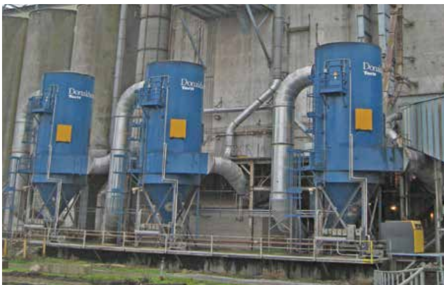
RF - Grain Terminal 61,000 cfm (103,618 m 3 /h)
