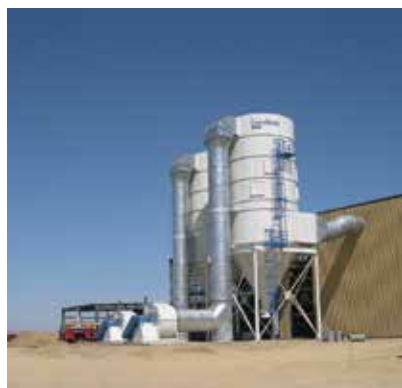
LP on Nut Dust 280,000 cfm (475,622 m 3 /h)
