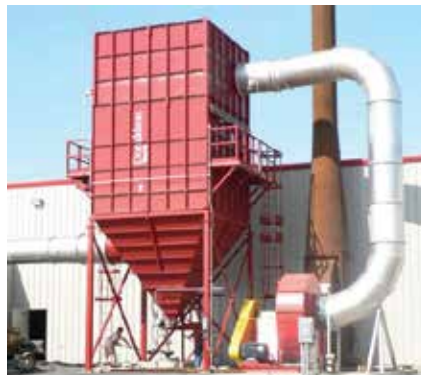
MB on Glass Processing 25,000 cfm (42,466 m 3 /h)
