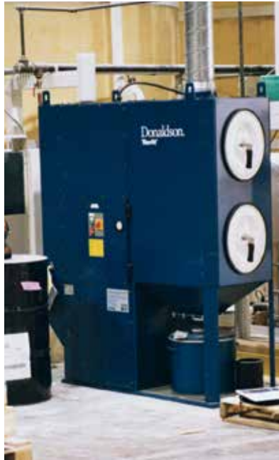
DFO on Paint & Pigment 1,200 cfm (2,038 m 3 /h)
